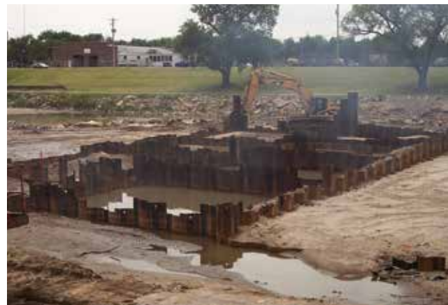
Permanent steel sheet pile grid utilized to take vertical load of Lincoln Street Bridge and Dam in Wichita, Kansas.
