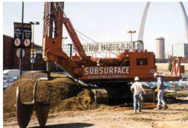
Cleaning out drilled shaft casing in St. Louis, MO.
