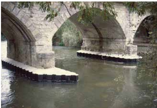
Permanent steel sheet pile cofferdam used as form work, and scour and impact protection.
