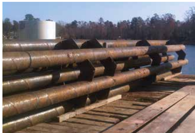
Reinforcement cage made with spiralweld pipe. Additional threaded bars installed inside pipe.
