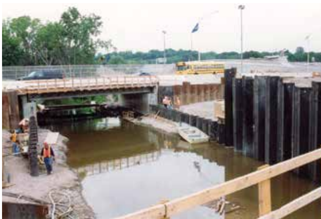
Sheet piles carry full load of bridge in Paramus, NJ.
