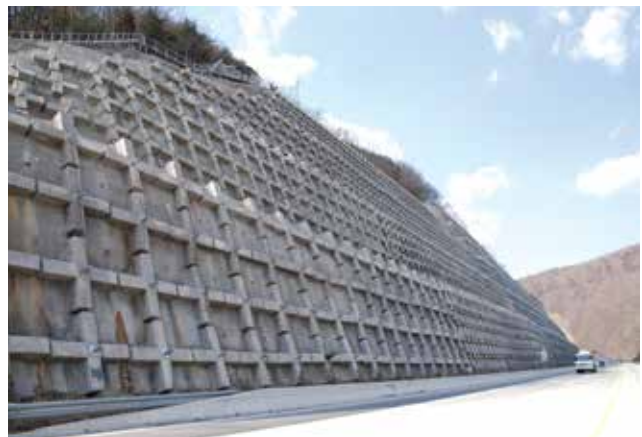
Slope stabilization with grouted soil anchors.
