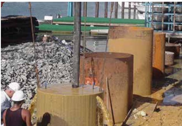
Pumping concrete for drilled shafts in Puerto Rico.
