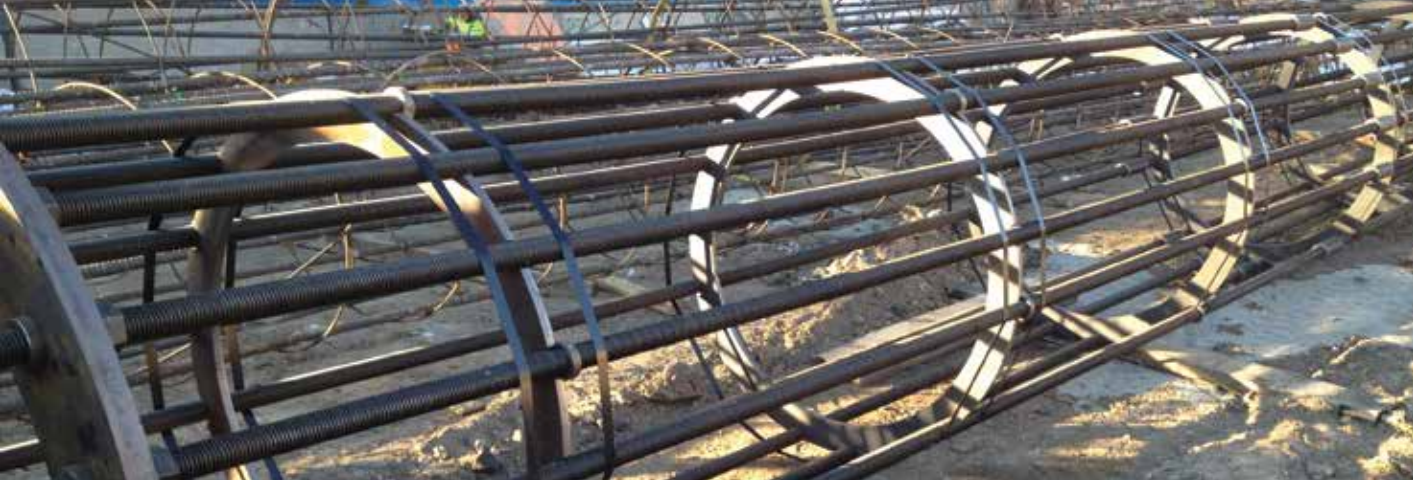
18 #18 grade 75 threaded bars for 72" drilled shaft in Minnesota
