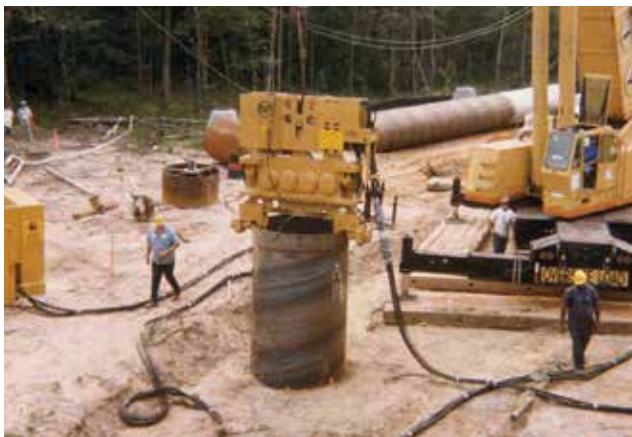
Installation of casing for drilled shaft.
