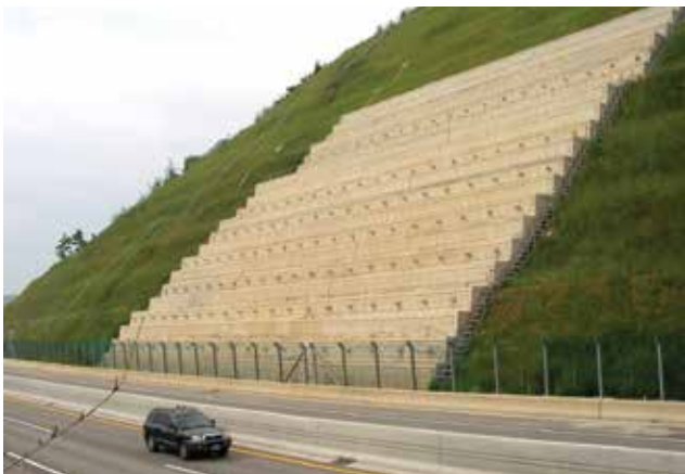
Slope stabilization with grouted soil anchors.
